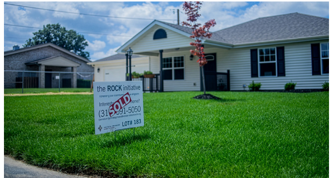
This single-family house in Arlington Woods in Indianapolis, Indiana, was built through partnerships made possible, in part, by the Neighborhood Program.
