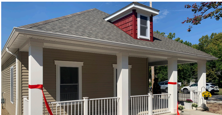
Thirty units of affordable housing were developed in the Buckeye-Larchmere neighborhood of Cleveland through partners brought together through the program. Thirty single-family homes were built for families at or below 60% of the area median income. Through CHN Housing Partners, the homes were rented on a lease-purchase basis with the goal of residents being able to purchase the homes from the developer after 15 years.
